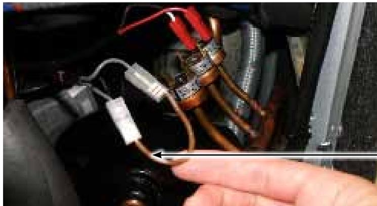
The image shows bridging on the operating pressure switch
