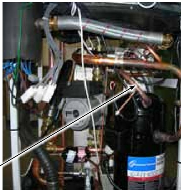
The discharge pipe must be hot (not lukewarm) even slightly away from the compressor if the phases are in the correct sequence.
