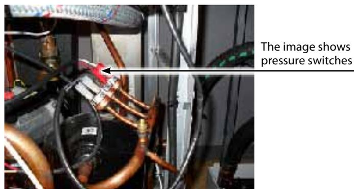
**The operating pressure switch does not open but the heat pump opens at high pressure**
