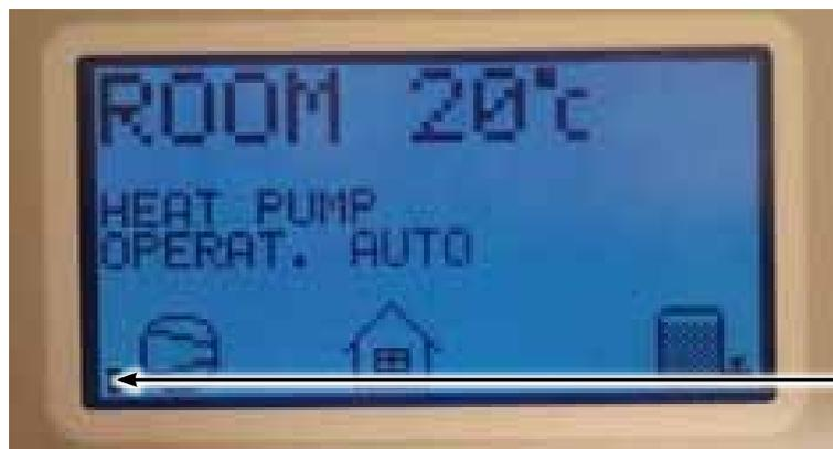
The image shows an open operating pressure switch or too high discharge pipe temperature
