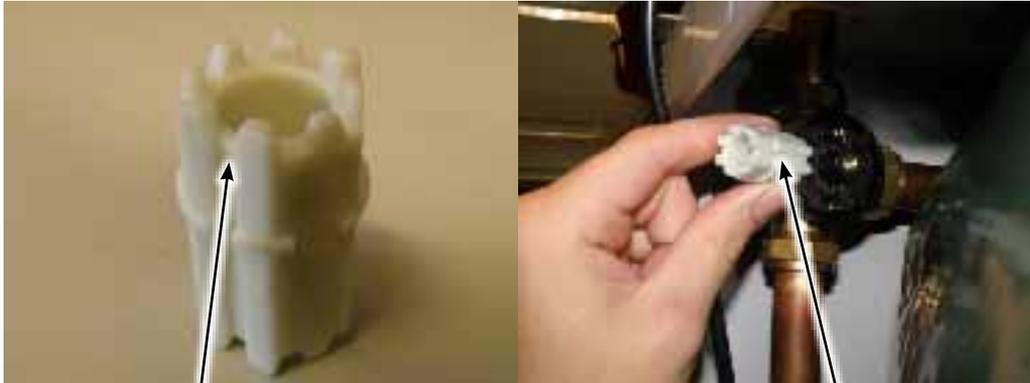
The groove of the white six edged sleeve must be towards 3 o'clock in unaffected mode.
